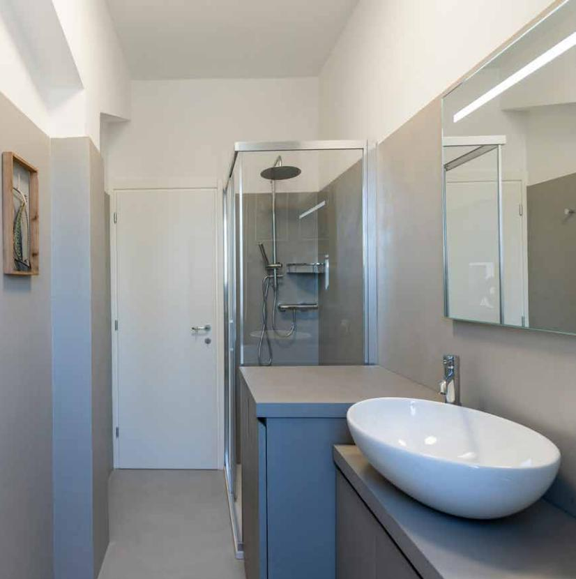
**EN** – Ideal Skin is used to create continuous and seamless surfaces on floors, walls and solid furnishings with an elegant, discreet and homogeneous design. It is applied by spatula in two coats with a total thickness of about 1,5 mm and is available in 16 basic colours that offer countless combinations.
